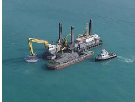
Backhoe with barge
