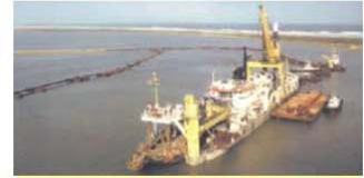
CSD with pumping ashore
